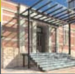
*A new entrance forecourt to the ballroom was created providing an identifiable entrance hall and space for open air assemblies. The new elements that make up the entry are a steel and glass stair and entrance canopy. Materials selected were distinctively contemporary to distinguish from original fabric.*
