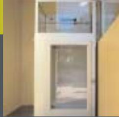
*A new glazed lift was installed to provide access to all levels and was designed to have the least visual impact and to disturb as little significant fabric as possible.*
